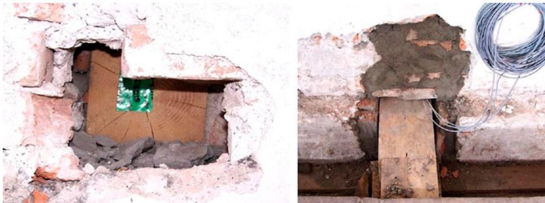
Figure 9. Variant N4/4b with fresh mortar in direct contact to the beam head (left) and. variant N5/3 with a lot of built in mortar (right). Photos: Fraunhofer Institute for Building Physics IBP.
