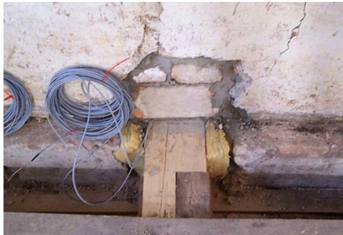
Figure 2. Variant 1 with common halving, mortar bed and insulation mounted around the beam head. Photo: Fraunhofer Institute for Building Physics IBP.
