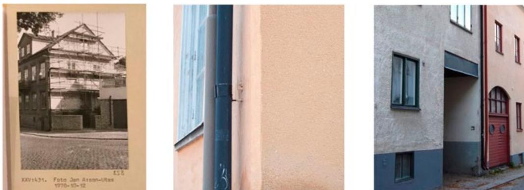
Figure 1. Two measures to exterior of houses derived from the EBB: additional façade insulation in *Berget 16* (left and middle) and additional insulation of the system of joists (right). Photos: Mattias Legnér.
