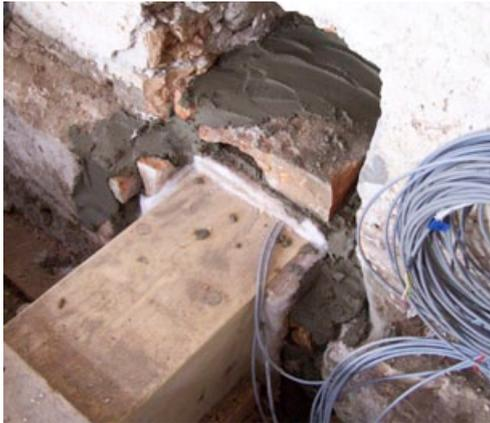
Figure 4. Variant 5 with common halving, aerogel mat around the beam head and as support. Photo: Fraunhofer Institute for Building Physics IBP.
