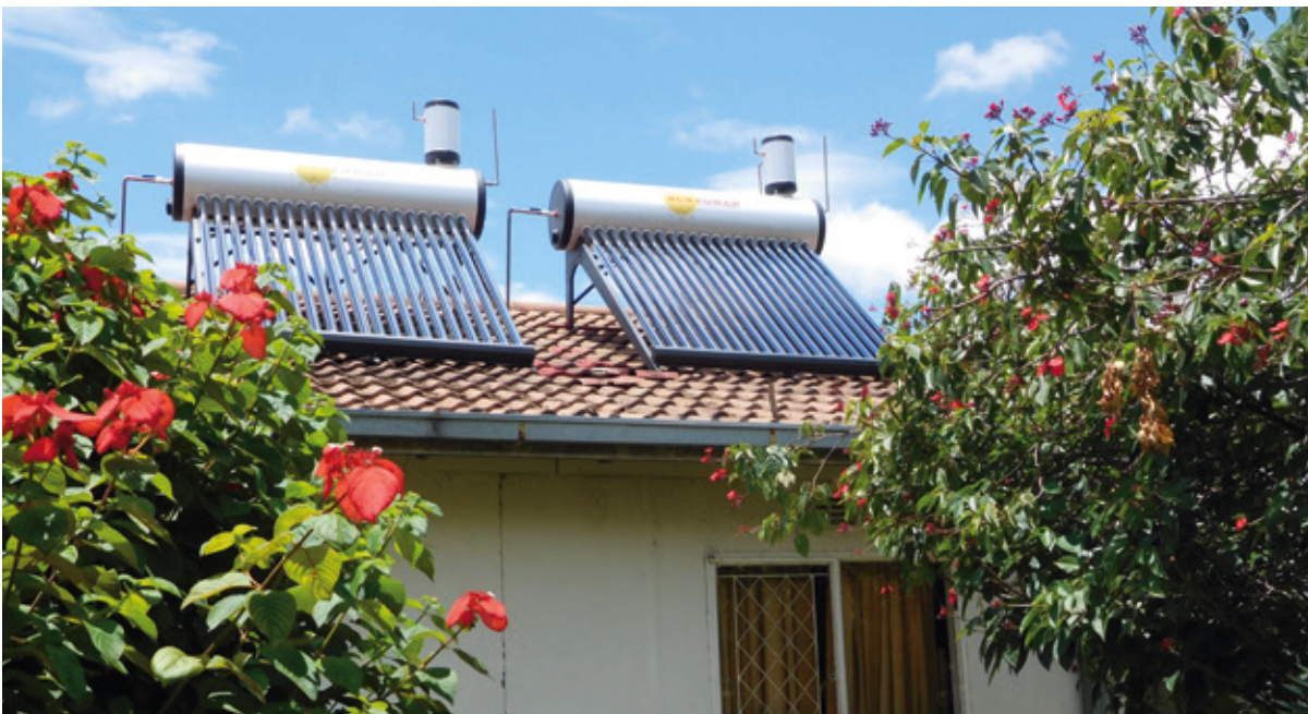
Thermosiphon systems at the CPS Sisters youth hostel in Harare, Zimbabwe Photo: Werner Weiss, AEE INTEC
