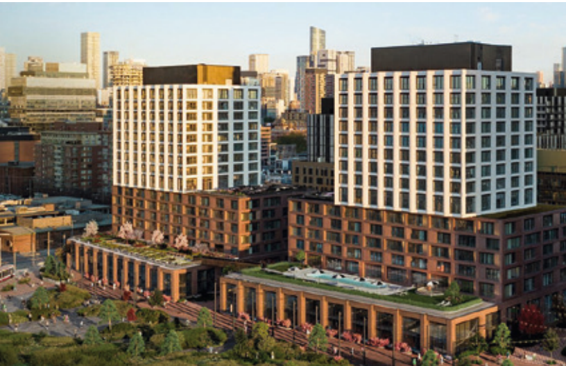
Solar air heating systems on the mechanical room penthouses at the Canary Commons, a condo community in Toronto, Canada Photo: SolarWall Conserval Engineering Inc.
