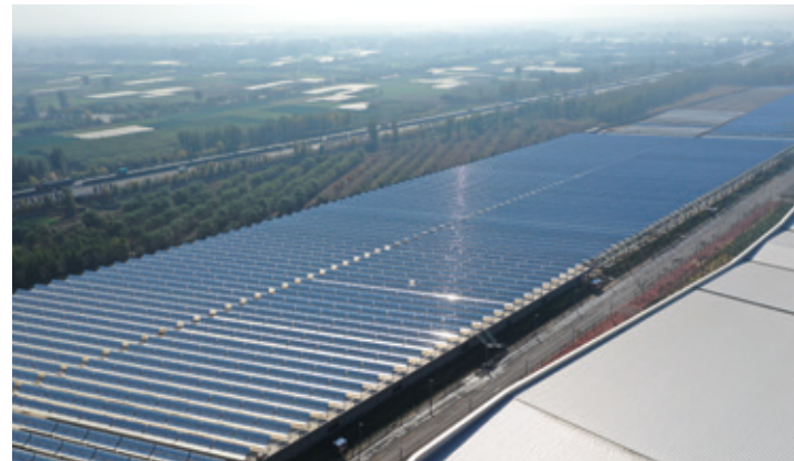
An 80 MW th parabolic trough collector system supplies snow for an indoor ski hall, as well as heating and cooling at the Handan Bay Water World in China
