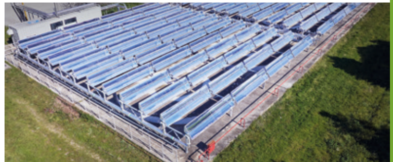
Parabolic trough collectors for one of the breweries of the Carlsberg Group in Salonika, Greece
