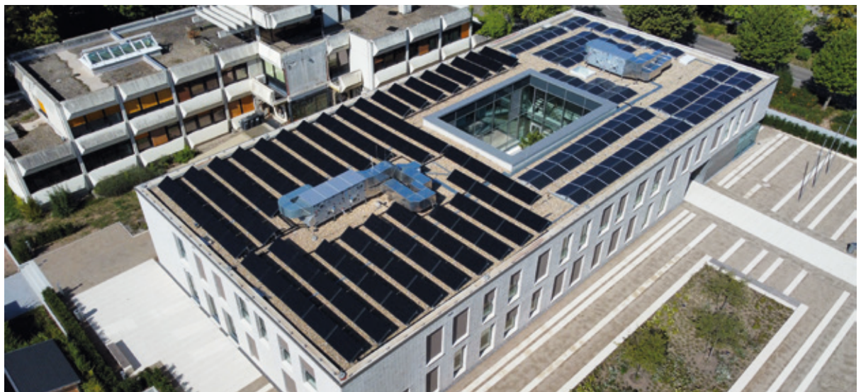
100 PVT solar panels at the town hall Offenbach an der Queich, Germany, operate in combination with a 50 kW heat pump
