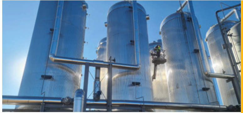
Heat storages for the Heineken brewery in Seville, Spain Photo: Engie, Spain
