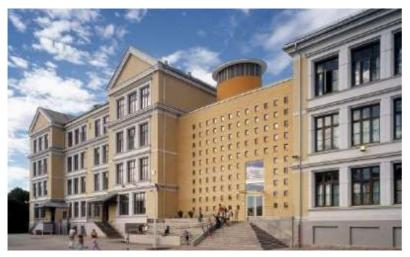
The building envelope of the *Kampen School in Oslo* was kept as built, but a new building was built between the two existing buildings. By doing this, the energy demand per square meter of the surface area for the total school building was reduced.
