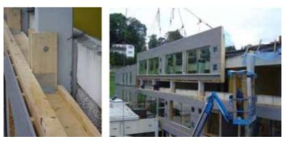
Figure 8 School in Schwanenstadt: installation of facade elements
