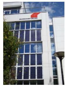
Figure 17 Façade integrated PV system, Office Building Roskilde
