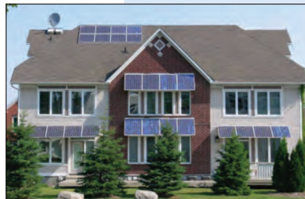
Candian Centre for Housing Technology in Ottawa, Canada.
