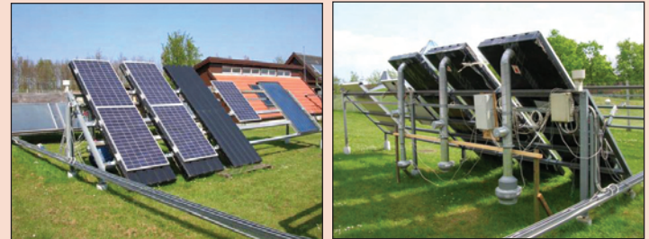
Front and back views of two SolarWall® PV/T transpired air collectors, one thermal reference and one PV reference in the test stand at the Danish Technological Institute.
