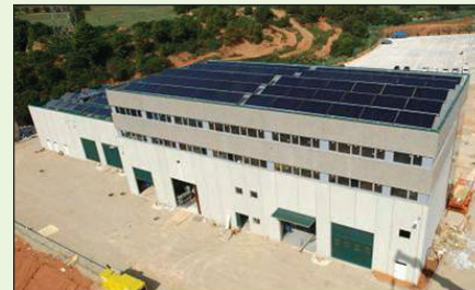
Contank plant for container washing, Barcelona, Spain. Installed capacity: 357 kWh.
